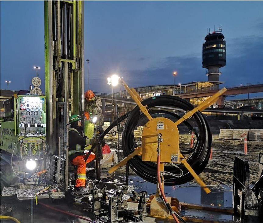
The Memorandum of Understanding between PPI and IGSHPA will advance the benefits that both organizations provide to the geothermal exchange industry. This geothermal system at Vancouver International Airport (YVR) used 841 single U-bend geothermal loops, each 1,000 feet long, with a molded and heat-fused U-bend installed at the mid-point. Image Courtesy Versaprofiles
